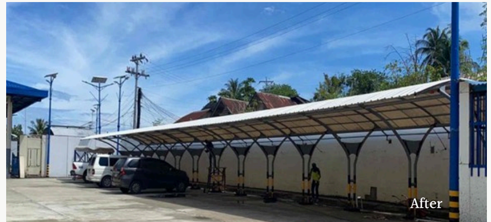
Maintenance of Parking Area at POB Complex, Nasipit Port
